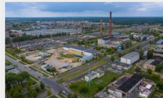
PUBLIC INFRASTRUCTURE DEVELOPMENT OF THE NORTHERN INDUSTRIAL ZONE OF DAUGAVPILS CITY, PHASE III
